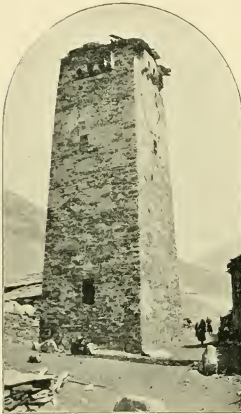
A TOWER AT USHKUL
